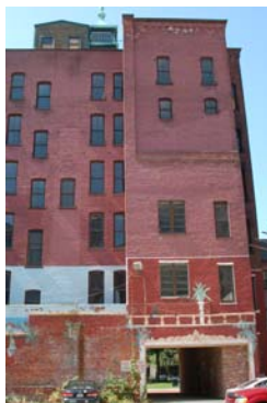
STATE ST. VIEW THROUGH ORIGINAL ENTRY
